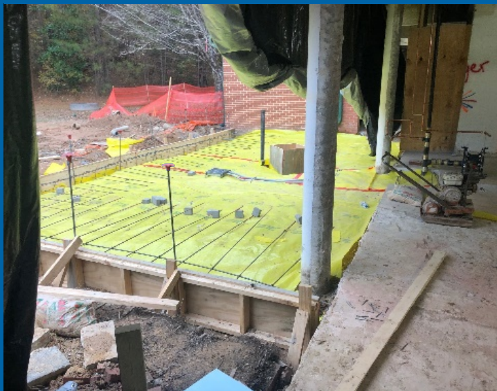
Admin Addition SOG Prepped for Concrete
