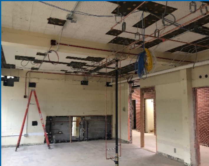
Plumbing and Electrical OH Installation at SW Wing
