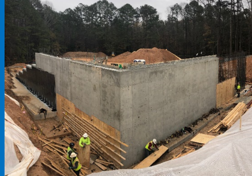
Continuation of Wall Pours at Gym Area
