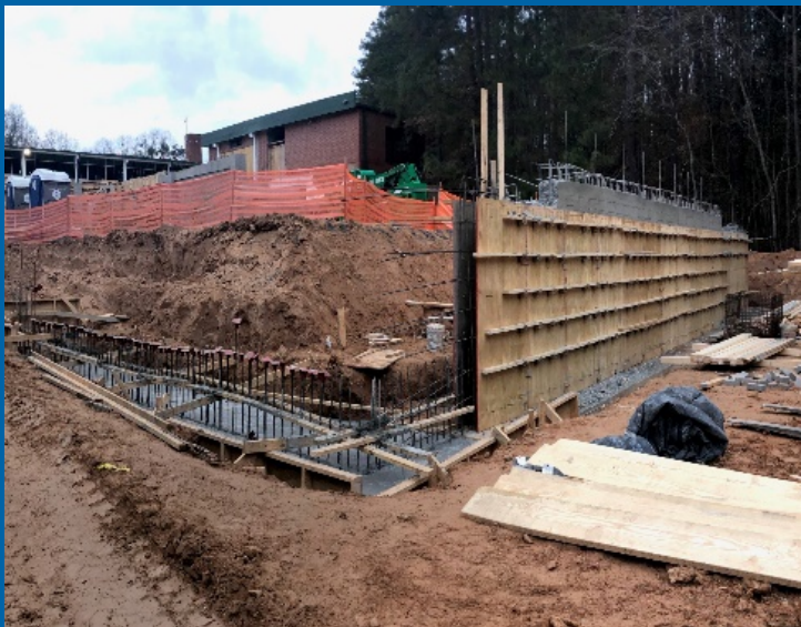
Gym Addition North Wall and Footing Concrete Pour
