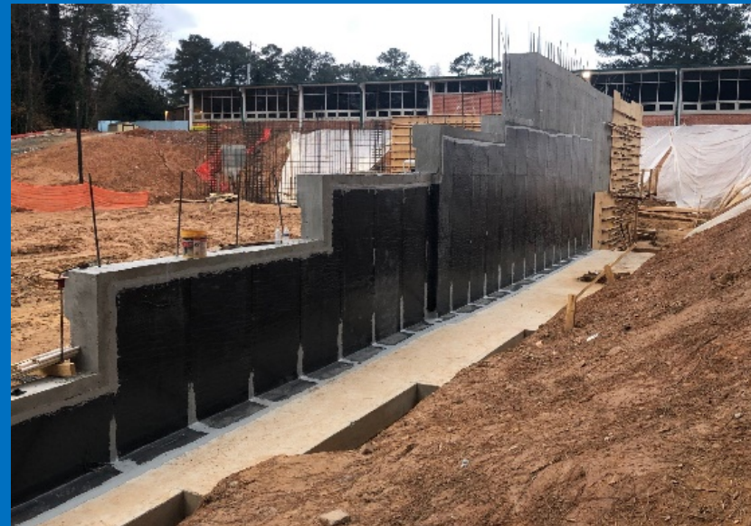
Waterproofing Installation at Gym Area
