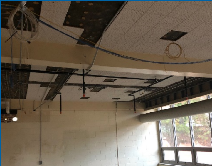
Fire Protection OH Installation at SW Wing
